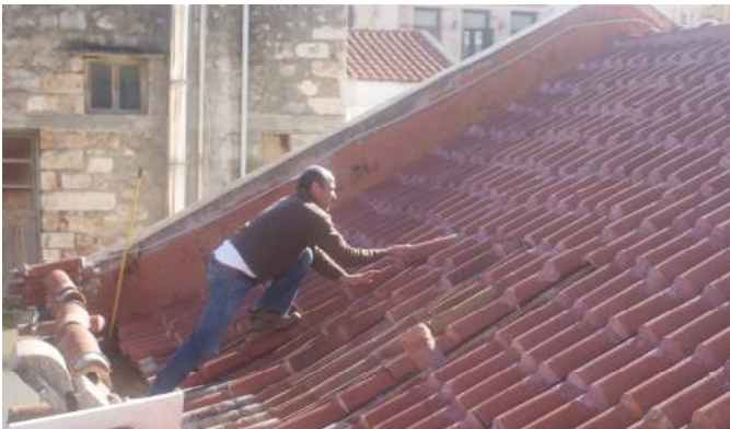
Maintenance works on the northern roof of Etz Hayyim.
