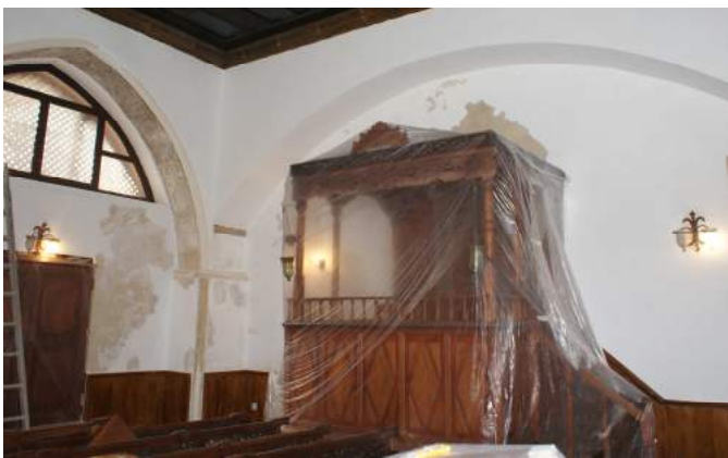
Renovation works, Etz Hayyim interior, February 2016
